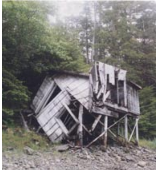
Ruins of one of the Thompson buildings in Greentop Harbor in 1994.
